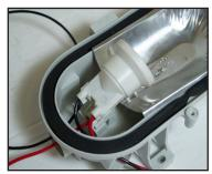
Once the deisred number of wires are connected to the bulb recepticle, snap the wired recepticle into the fixture's base. Screw a properly sized bulb in the socket (see page 1 for details). Install lens and guard.
