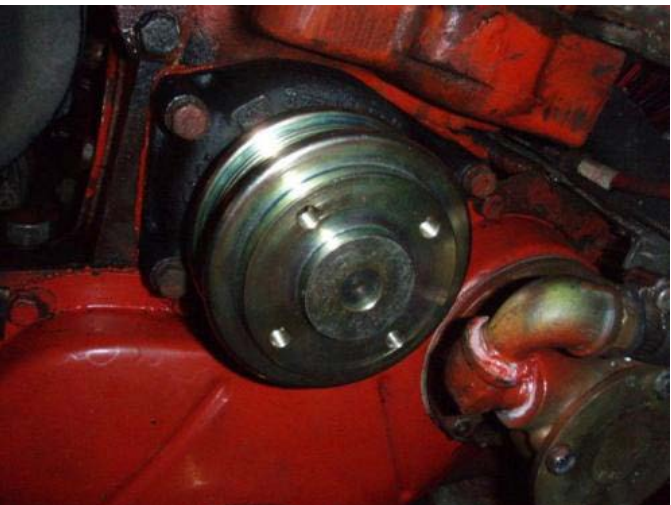
18. The new water pump shown installed on the engine.
